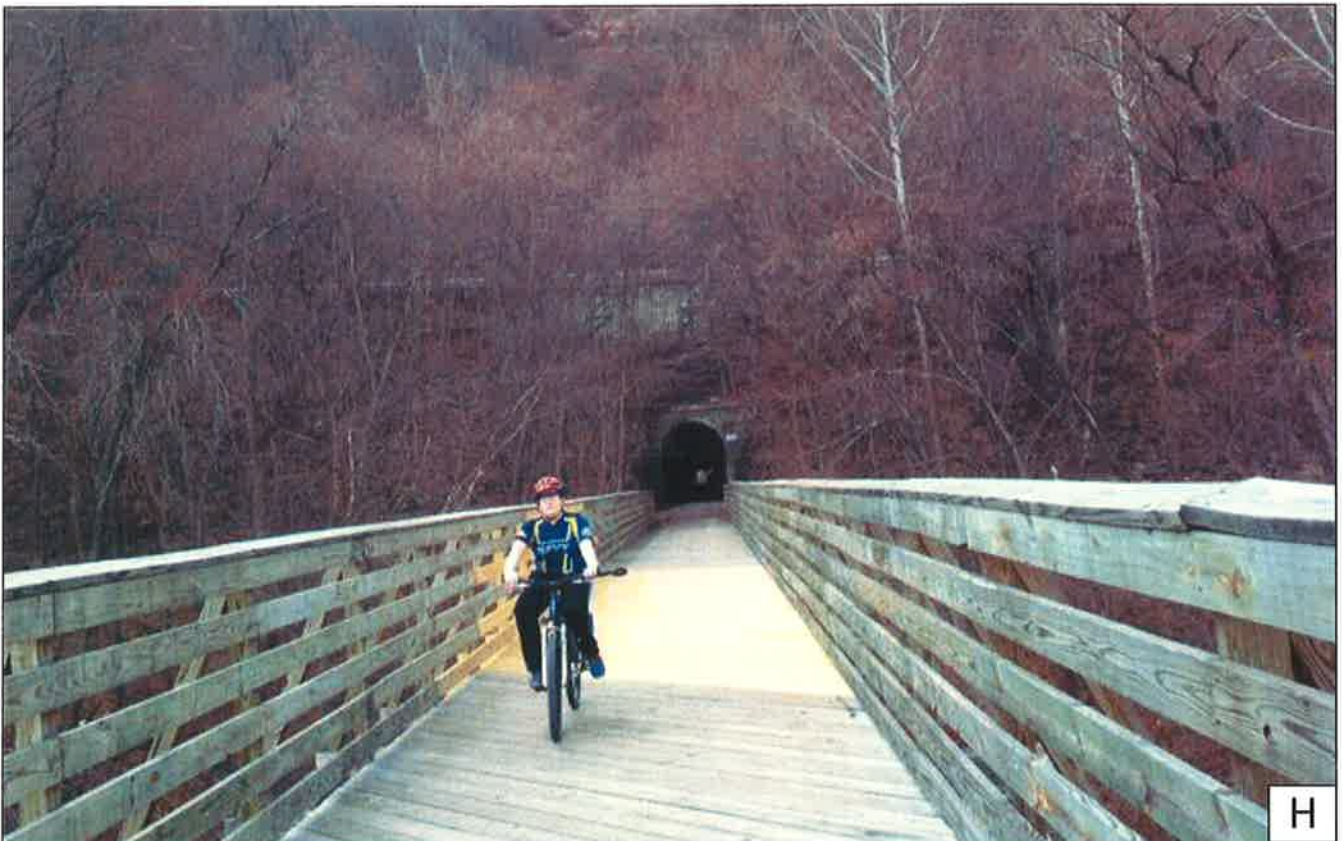
Carpendale trestle and tunnel
