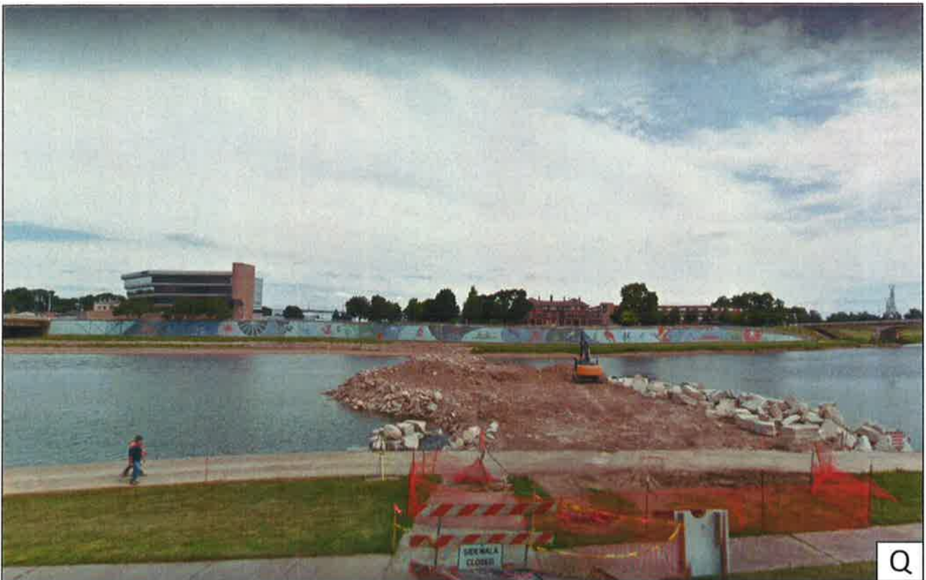
Drop feature under construction
