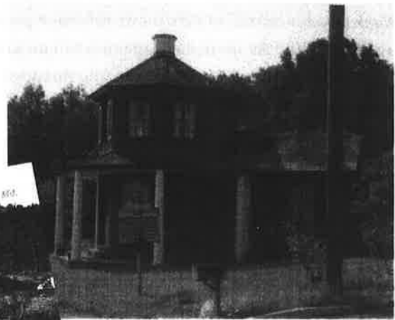
Figure 90: The LaVale Tollhouse, one of the few remaining tollhouses from the National Road, lies along the route from Cumberland to Frostburg. (WRT)
