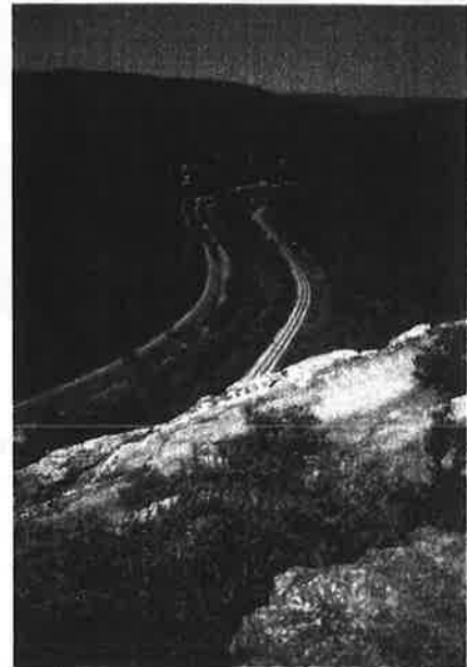
Figure 62: The present day landscape of the Narrows is shared by the CSX (B&O) railroad's main line track, the WMSR's excursion line right of way, and US Alternate Route 40. Sandwiched between these routes is Wills Creek and a "scenic" automobile pull-out. The combination of local, county and state interests should move to establish a long-term management program that safeguards this scenic and historic landscape.
