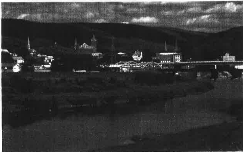
Figure 55: A panoramic view of the church spires and courthouse tower of Cumberland's west side will greet visitors entering Cumberland on the proposed Canal Parkway. While easily taken for granted, the charm of the nineteenth century architecture and dramatic mountain setting of the city is most compelling to visitors, a fact that was strongly emphasized by respondents in market research focus groups. (MSHA)
