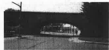
Figure 57: The limits of the Preservation District, defined by state legislation, were established by examining logical physical boundaries, such as the B&O Rail viaduct along Queen City Drive. (WRT)
