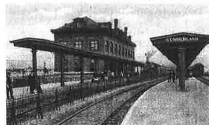
Figure 64: Surrounded by Station Square and the Wills Creek Promenade, the Western Maryland Railway Station will be the orientation point for visitors to Canal Place. The Station will include a new NPS Visitor Center with interpretive exhibits, Western Maryland Scenic Railroad ticketing and offices, and offices for the Canal Place Authority, NPS, and the Allegany County Visitor's Bureau. (Al Feldstein)
