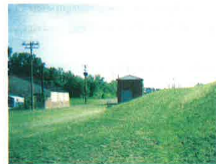
Figure 27: The Mill Race Pump Station is the focus of an extensive network of subsurface utilities, some of which will require relocation to enable the canal rewatering in the Terminus. (WRT)
