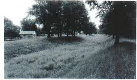
Figure 16: The shape of the C&O Canal prism is illustrated in this view of the existing canal bed in South Cumberland. (WRT)
