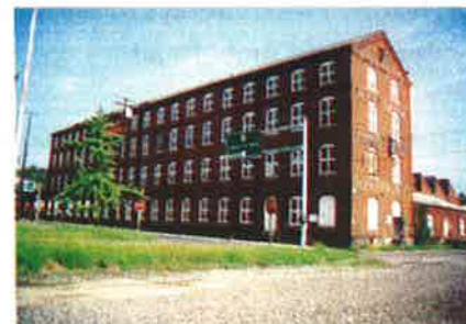
Figure 23: The remaining buildings of the Footer’s Dye Works complex offer an opportunity for adaptive re-use for heritage-related uses. (WRT)
