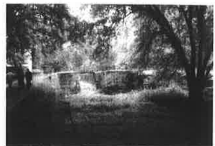
Figure 71: The stone structure of the lift locks at North Branch is suitable for restoration of operating lift locks. The image and experience of the actual operation is an invaluable interpretive tool in describing the engineering aspects of canal operation. (WRT)
