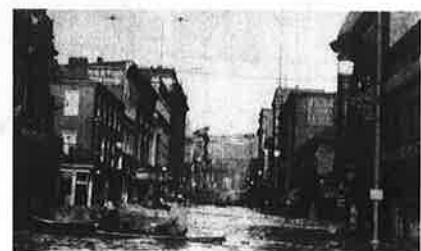
Figure 52: The 1924 flood provided enthusiastic canoeists with a chance to shoot the rapids on Baltimore Street. Floods such as this accelerated the decline of the canal, as the expense of maintaining the fragile canal system outstripped the canal's profitability. (Al Feldstein)
