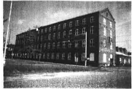
Figure 99: The remaining structure of the Dye Works is a four story brick loft-style building. (WRT)
