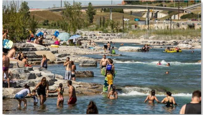
Stone terracing and river access at a dam modification project in Calgary, Alberta.
