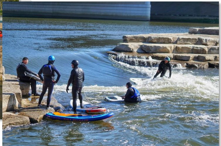
A casual river surf scene at a dam modification project in Dayton, Ohio. This surf structure shown is anchored directly to a defunct low-head dam.
