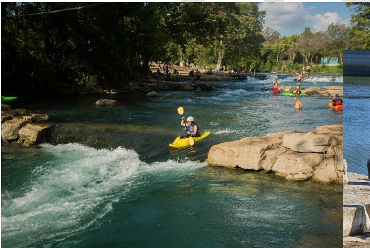
A beginner kayaker descends a recreational drop structure in San Marcos, Texas designed by REP. These structures perform together with, and are anchored to a defunct mill dam, a common site scenario and opportunity for river recreation.
