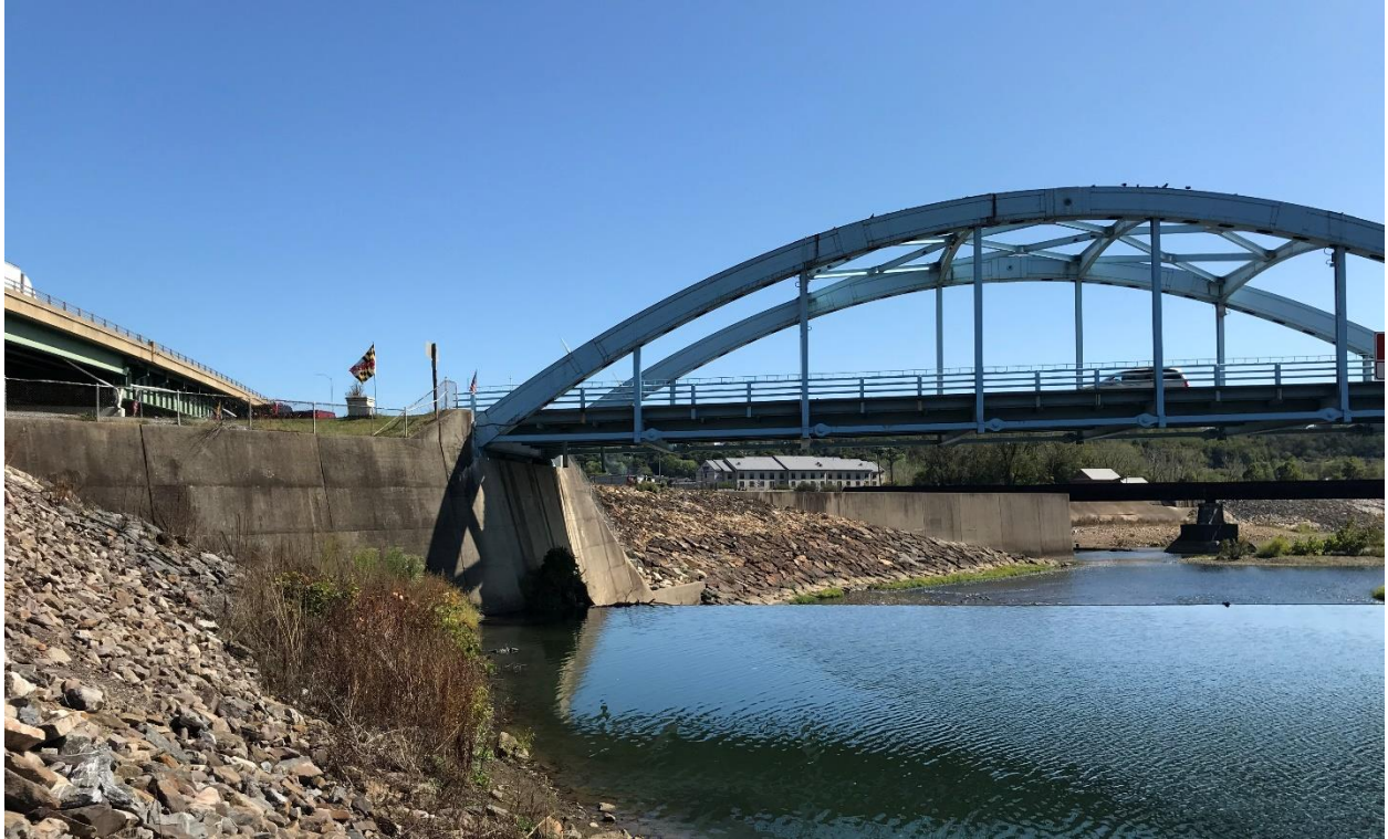
Existing floodwall and dam on river left (Maryland). Proposed location of trail underpass adjacent to feature whitewater drop.
