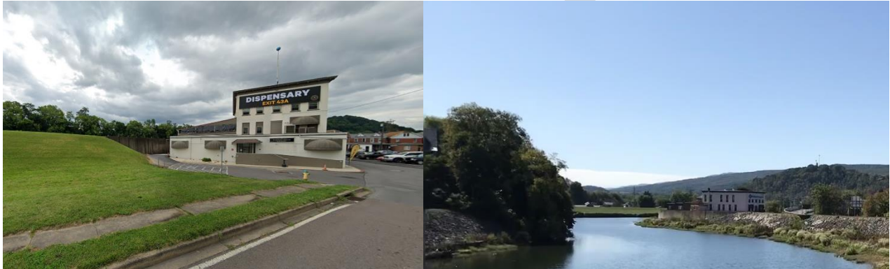
Existing Aviertt Street floodwall and Levee. Proposed whitewater launch point.
