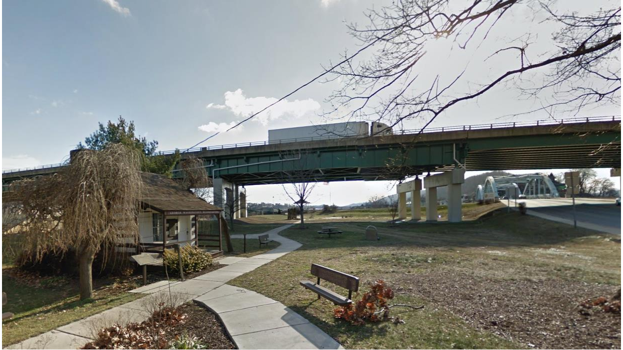
Existing Riverside Park includes National Road 0-mile marker, George Washington's Headquarters. Proposed location of parking lot access for take-out location for whitewater park and the relocation of George Washington's Headquarters to the point of the Riverside Park.
