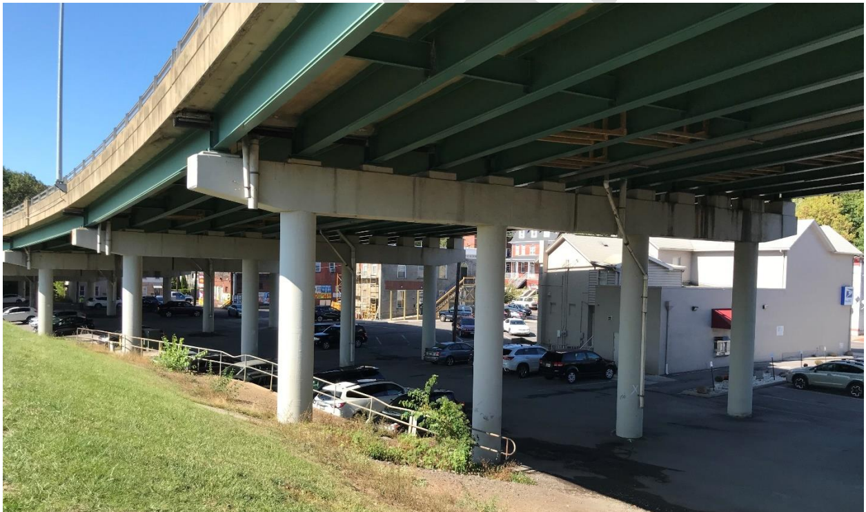
Existing Interstate 68 Bridge parking lots on Greene Street. Proposed area of shared use parking for the river park.
