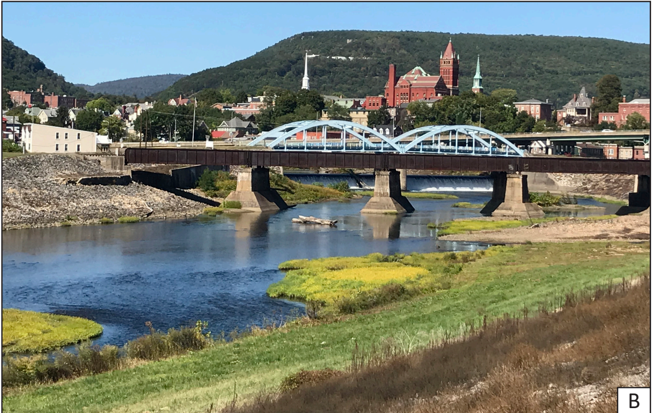
Drop feature #4 area facing upstream
