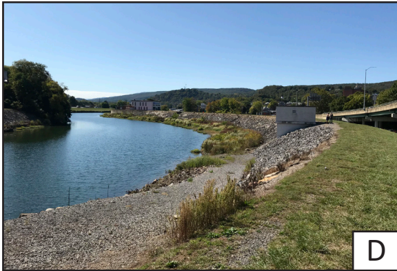
Feature drop #1 and water intake area
