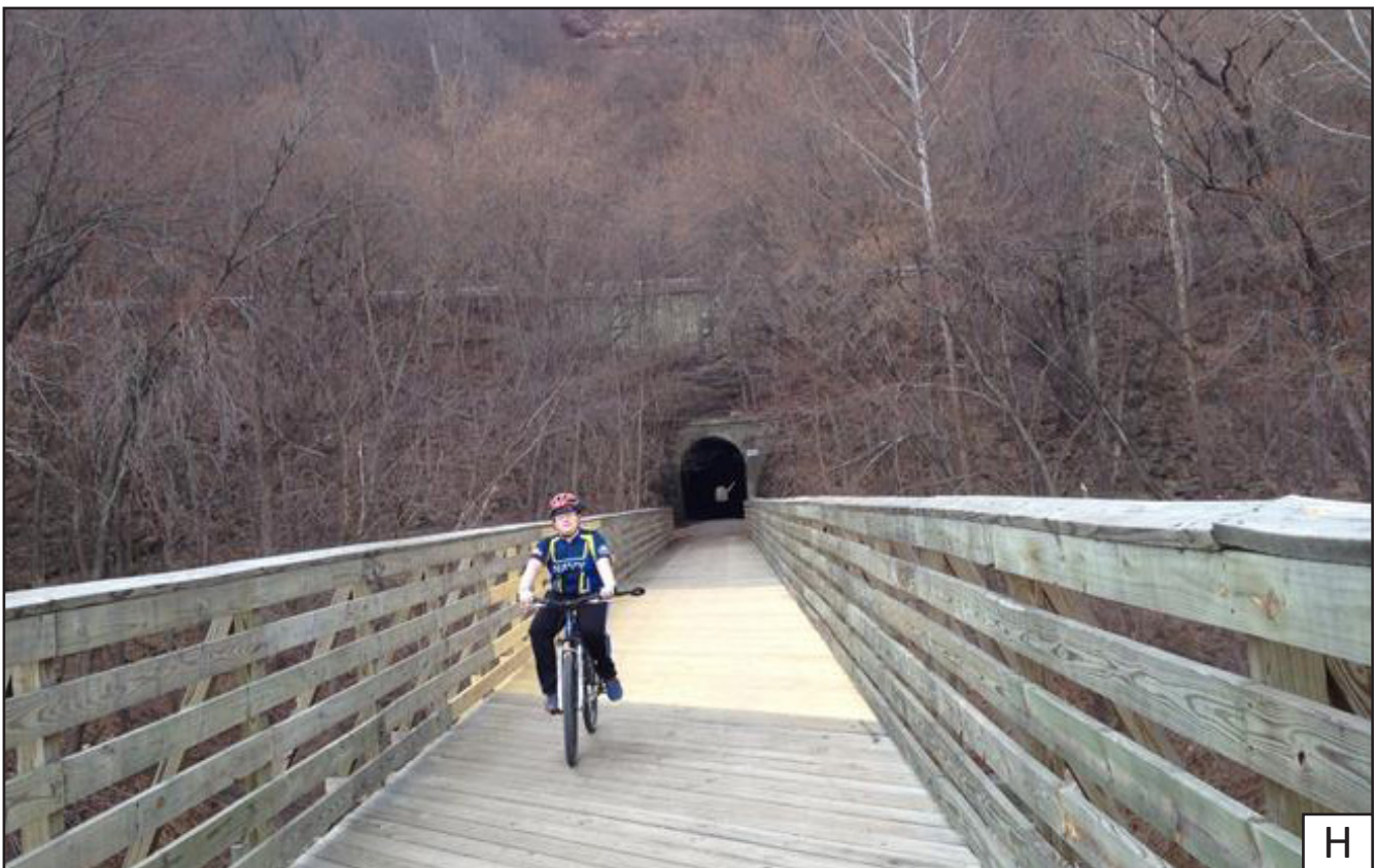
Carpendale trestle and tunnel
