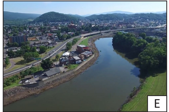
Upper pool area facing downstream
