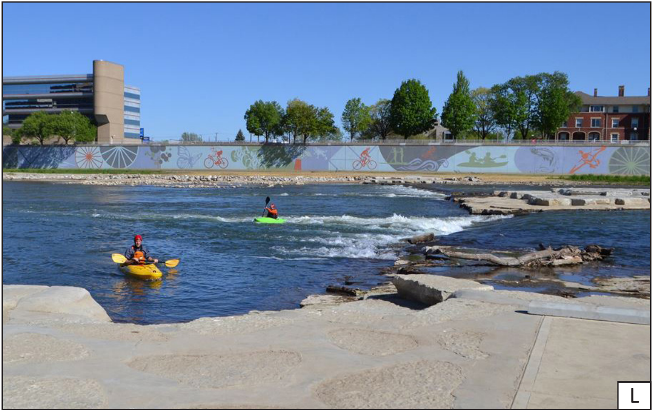
Former dam site with drop features and murals on flood wall
