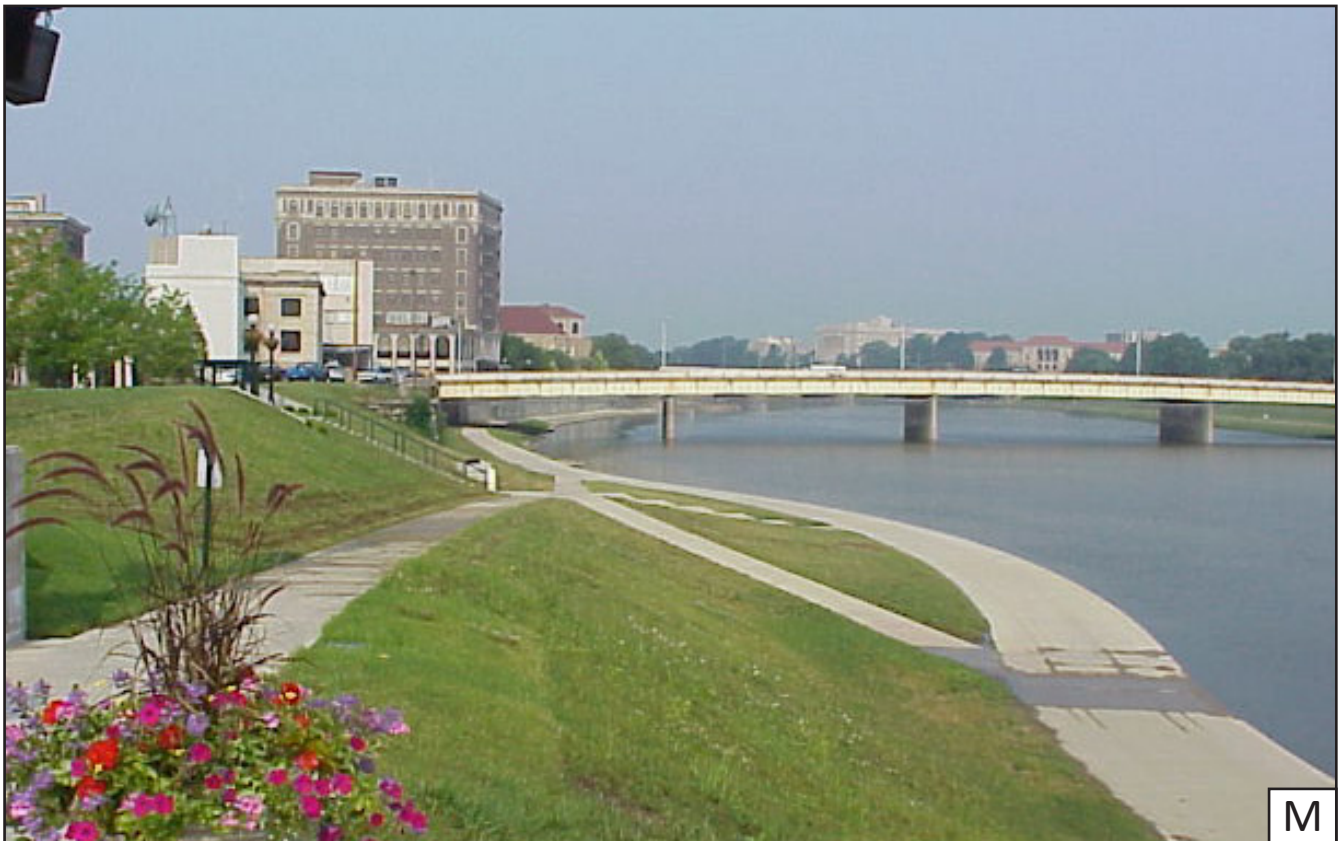
ADA access and multi-use concrete trail
