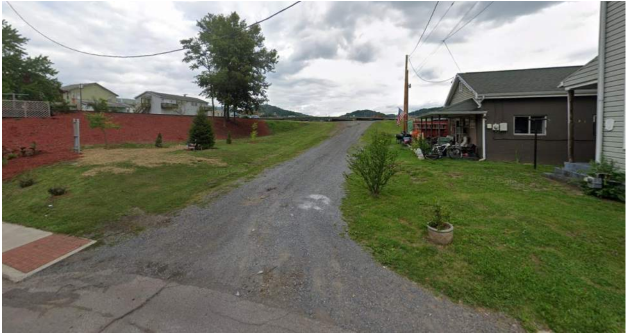
Existing gravel access to overhead electric lines on WV-28 Veteran's Memorial Highway. Proposed asphalt turnaround with parking for downstream of river park boat launch points and access to the trail network from the Ridgeley, WV side of the North Branch of the Potomac River.
