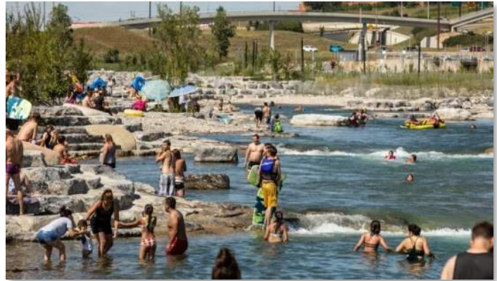
Stone terracing and river access at a dam modification project in Calgary, Alberta.
