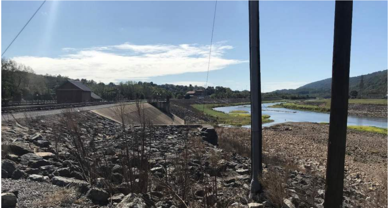
Existing flood wall River Left (Maryland side) downstream of railroad trestle. Proposed area for overlook and stair access to river trails.
