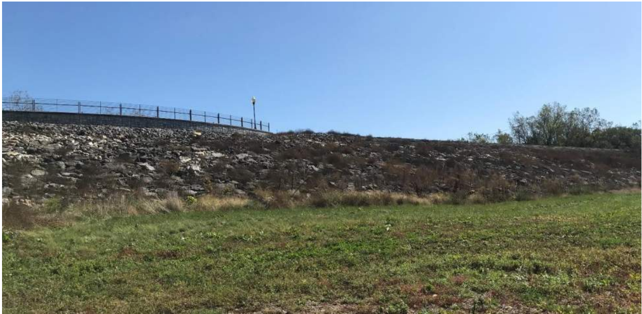
Existing overlook connected to the C&O Bike Trail. Proposed ADA access ramp to riverside trails.
