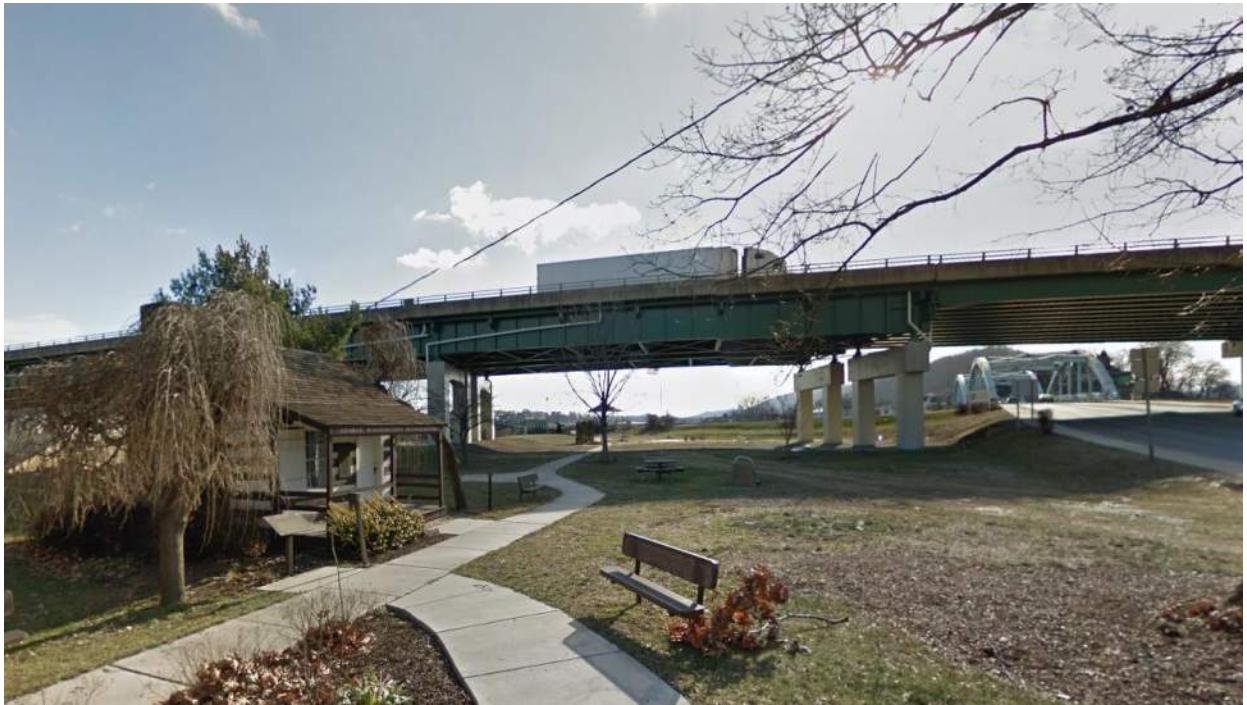
Existing Riverside Park includes National Road 0-mile marker, George Washington's Headquarters. Proposed location of parking lot access for take-out location for river park and better access to the Riverside Park.
