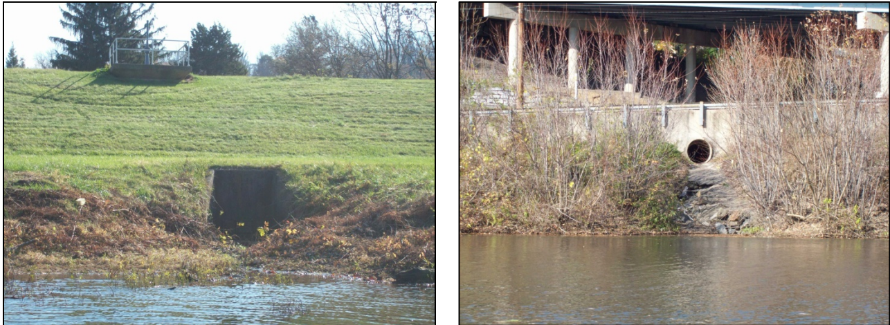
FIGURE 2. Levee drain outlet (a) and stormwater outfall (b) observed approximately 2,000 LF upstream of Cumberland Industrial Dam.
