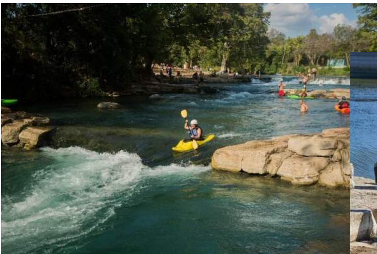
A beginner kayaker descends a recreational drop structure in San Marcos, Texas designed by REP. These structures perform together with, and are anchored to a defunct mill dam, a common site scenario and opportunity for river recreation.
