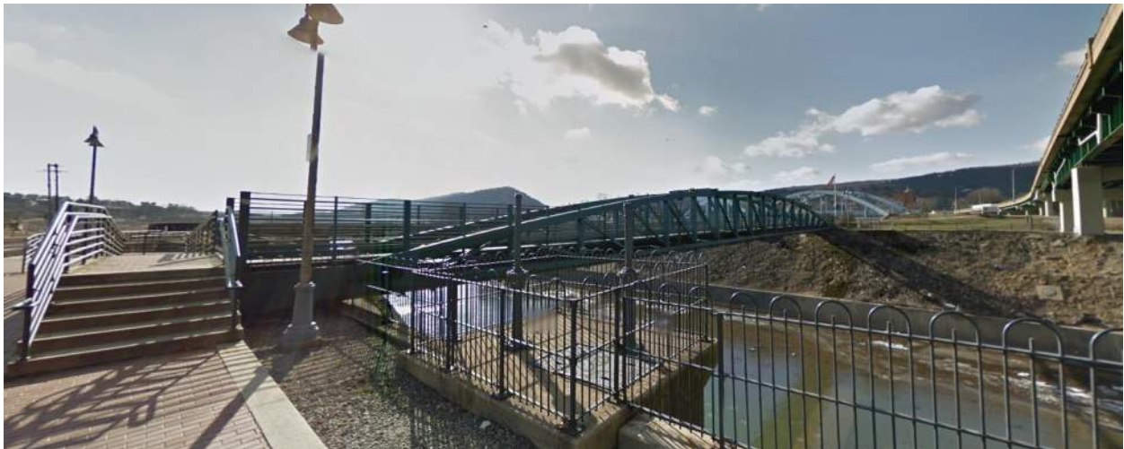
Existing Pedestrian Bridge with stairs and ADA access from Station to Riverside Park. Proposed connection point to Chesapeake & Ohio Bike Trail.
