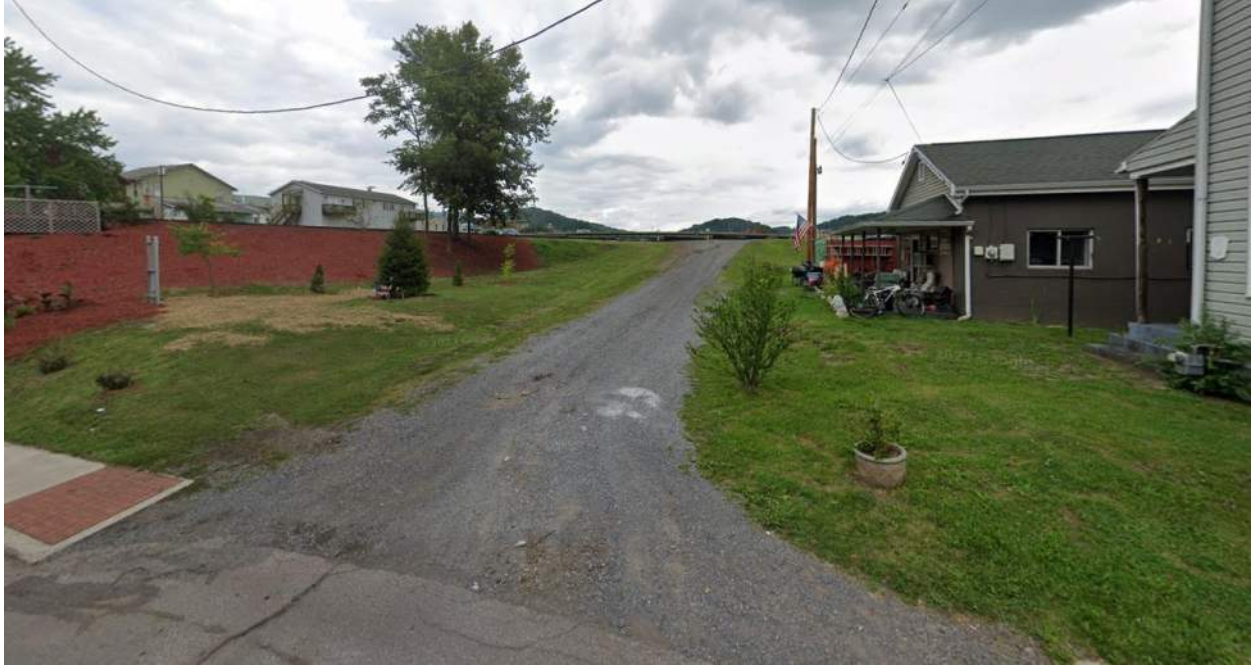
Existing gravel access to overhead electric lines on WV-28 Veteran's Memorial Highway. Proposed asphalt turnaround with parking for downstream of river park boat launch points and access to the trail network from the Ridgeley, WV side of the North Branch of the Potomac River.
