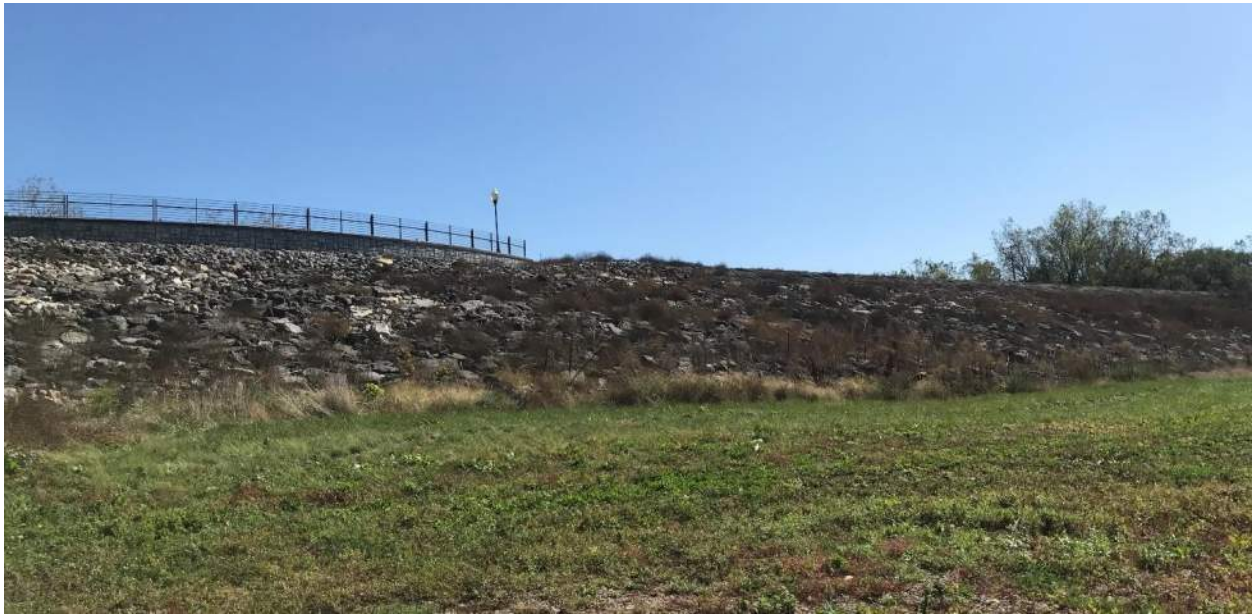
Existing overlook connected to the C&O Bike Trail. Proposed ADA access ramp to riverside trails.
