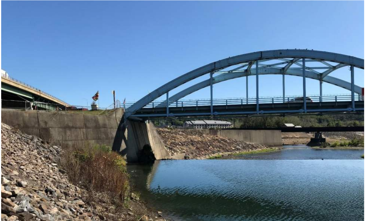
Existing floodwall and dam on river left (Maryland). Proposed location of trail underpass adjacent to water feature drop.
